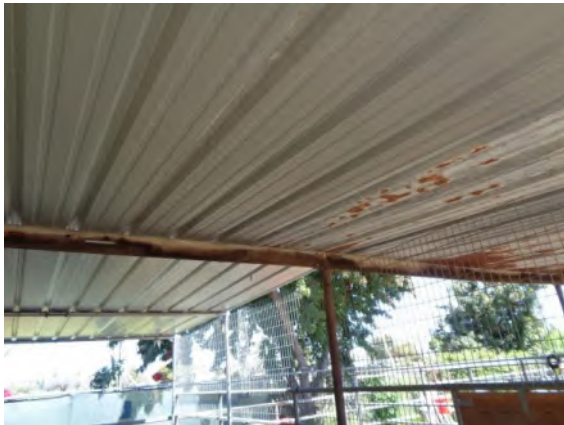
0042095a 4/2/2024 Corrugated metal expansion roofing with factory finish Stalls 142-146
