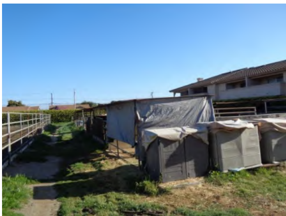
0042084a 4/2/2024 Boarding stalls with partial shade structure Stalls 152-158
