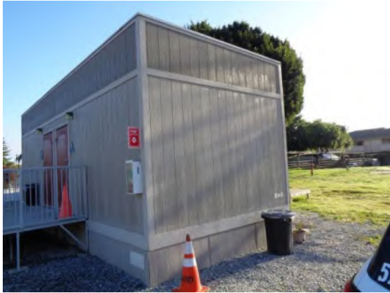
0042025a 4/2/2024 Painted T-111 plywood siding and skirting Restroom building, south elevation
