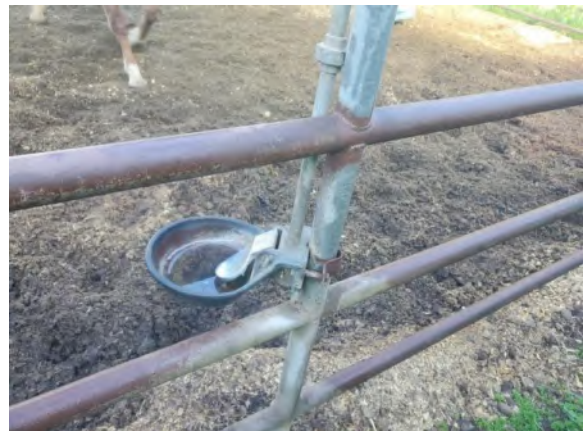
0042033e 4/2/2024 Galvanized steel pipe and steel waterer Stalls 159-169
