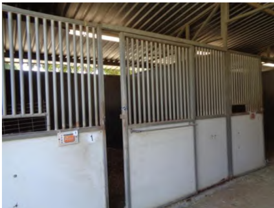
0042030a 4/2/2024 Sliding stall doors Barn 1-29 breezeway
