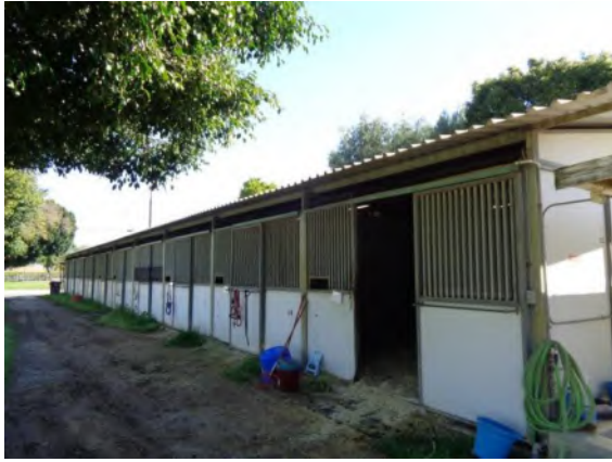
0042037a 4/2/2024 Exterior stalls with sliding stall doors Barn 1-29, west elevation
