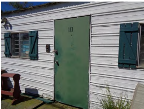
0042115a 4/2/2024 Typical door to tack shed with knob hardware Tack shed 10
