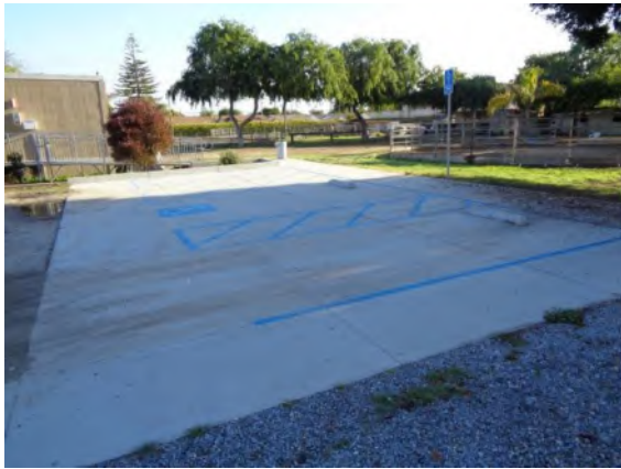
0042013a 4/2/2024 Accessible parking with concrete pavement and accessible routes to office and restroom buildings Between office and restroom buildings
