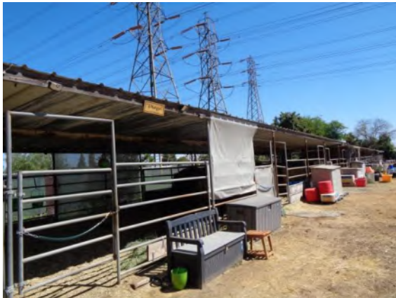
0042092a 4/2/2024 Boarding stalls with corrugated metal roof and pipe rail fencing Stalls 147-151
