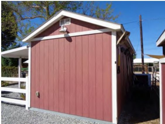
0042074a 4/2/2024 Painted wood siding of modular office Barnyard Buddies office
