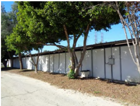
0042042a 4/2/2024 Composite metal clad wall panels Barn 1-29, east elevation
