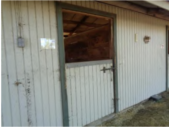
0042105a 4/2/2024 Wood exterior siding and stall door Stalls 170-172
