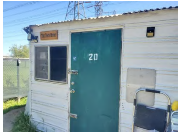
0042085e 4/2/2024 Overview of exterior systems Tack Shed 20
