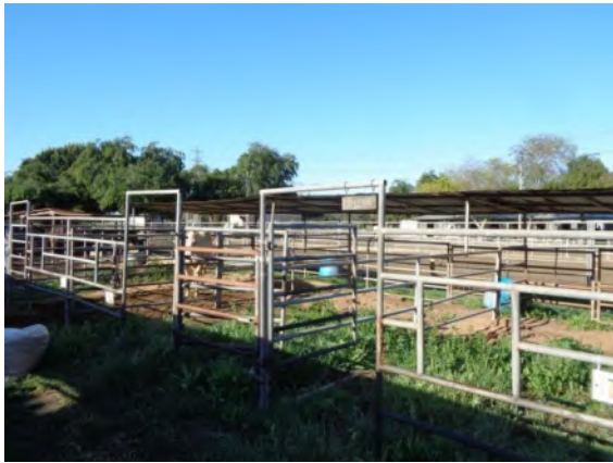
0042085a 4/2/2024 Pipe rail fencing of boarding stalls Stalls 152-158
