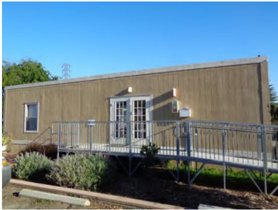
0042007a 4/2/2024 Painted T-111 plywood siding and skirting and metal entrance ramp and platform Office, south elevation
