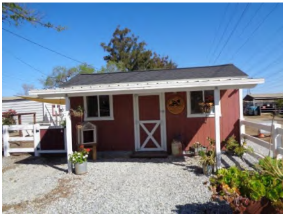
0042069a 4/2/2024 Modular office with asphalt shingle roof and corrugated metal canopy Barnyard Buddies office
