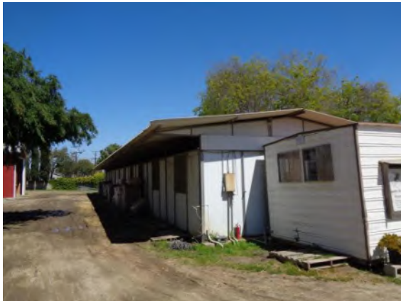
0042056a 4/2/2024 Corrugated metal roof, and painted, metal clad composite wall panels Barn 30-39, south and west elevations
