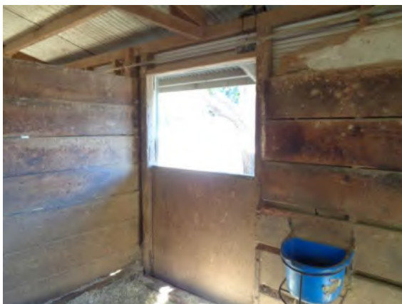
0042103a 4/2/2024 Typical stall door with OSB wood Stalls 170-172
