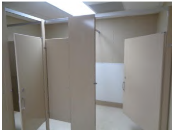
0042021a 4/2/2024 Painted metal partitions Restroom Building, men's restroom
