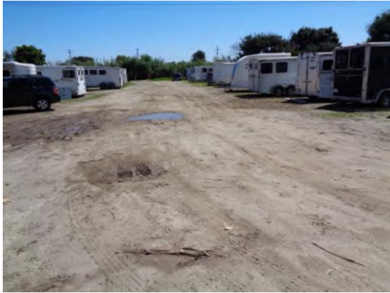
0042129a 4/2/2024 Dirt covered roadway with standing water Trailer parking area
