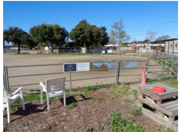
0042132a 4/2/2024 Standing water Arena E
