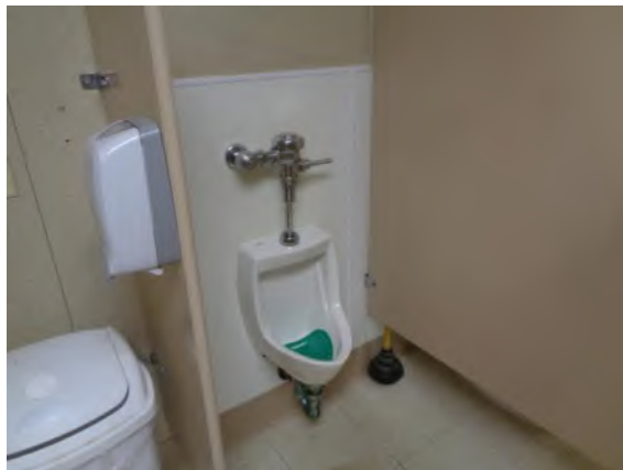
0042020a 4/2/2024 Urinal Restroom Building, men's restroom
