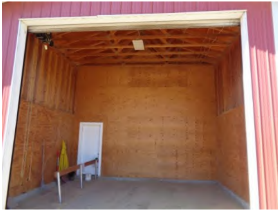
0042064a 4/2/2024 Hay storage room with unfinished wood walls Hay barn
