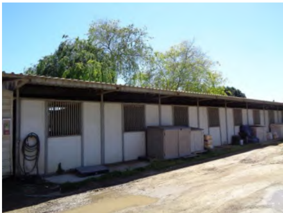
0042047a 4/2/2024 Corrugated metal roof and composite metal clad wall panels with fresh air grills Barn 30-39, west elevation
