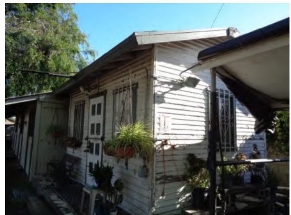
0042110a 4/2/2024 Wood siding on front and end walls Tack shed
