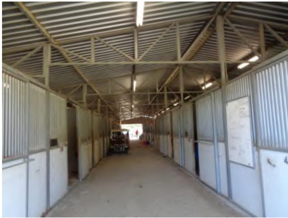
0042028a 4/2/2024 Corrugated metal roof and tubular steel frame Barn 1-29 breezeway
