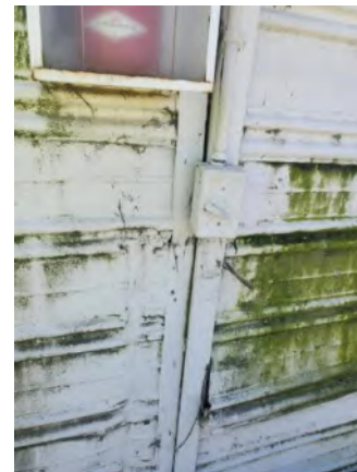
0042081e 4/2/2024 Aged electrical switch Tack Shed 11-12
