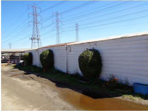
0042117a 4/2/2024 Corrugated metal exterior walls and roofs Tack sheds 9A, 9B, and 10
