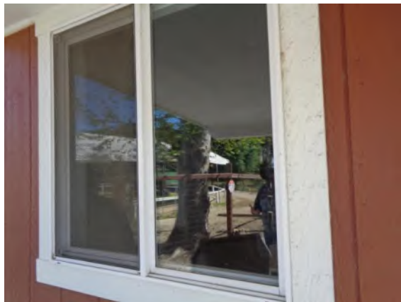
0042071a 4/2/2024 Office window with double-pane glass Barnyard Buddies office
