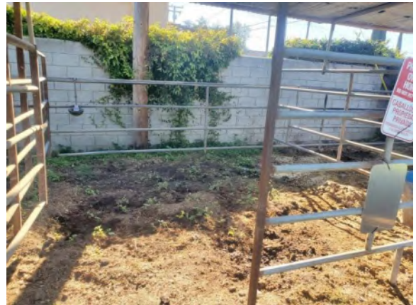
0042044e 4/2/2024 Galvanized steel pipe and steel waterer Stalls 173-180
