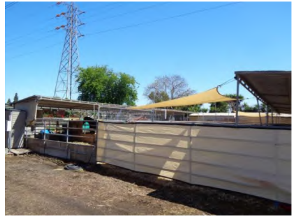
0042100a 4/2/2024 Boarding stalls with shade structures on either side Stalls 124-135
