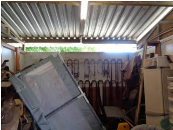
0042035a 4/2/2024 Stall 10 used as tack room Barn 1-29 interior
