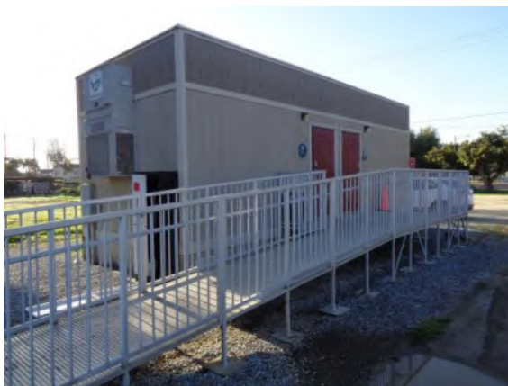
0042024a 4/2/2024 Painted T-111 plywood siding and metal access ramp with handrails Restroom building, west elevation
