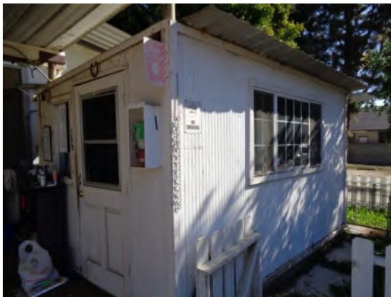
0042044a 4/2/2024 Wood storage shed with corrugated metal roof Barn 1-29, south elevation
