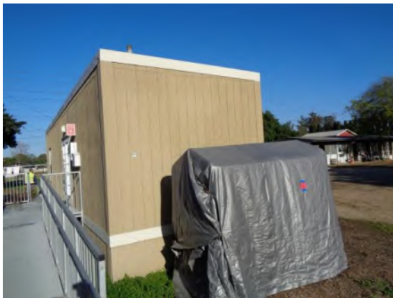
0042006a 4/2/2024 Painted T-111 plywood siding and skirting Office, east elevation
