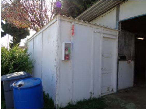
0042040a 4/2/2024 Wood storage shed with corrugated metal roof Barn 1-29, north elevation
