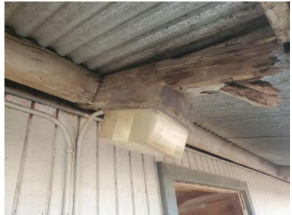
0042037e 4/2/2024 Surface mounted HID light Stalls 170-172
