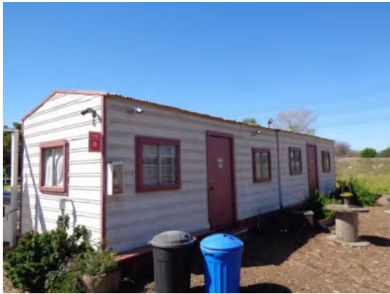
0042082a 4/2/2024 Metal sheds with corrugated metal roof and siding Barnyard Buddies
