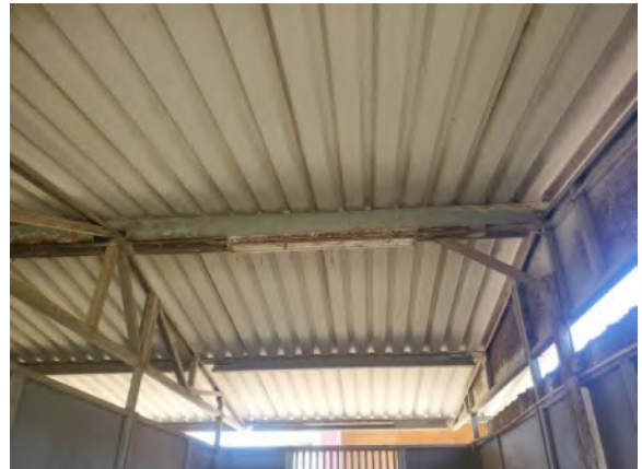
0042092e 4/2/2024 Surface-mounted lighting with T12 lamps Barn 30-39
