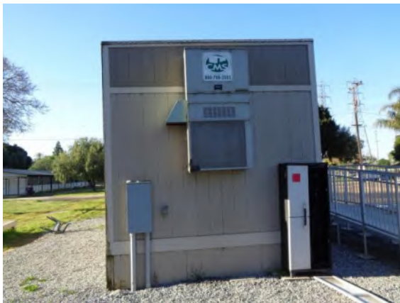
0042027a 4/2/2024 Painted T-111 plywood siding and skirting Restroom building, north elevation
