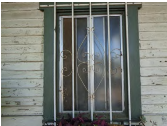
0042109a 4/2/2024 Single-pane glass window Tack shed
