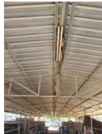
0042075e 4/2/2024 Overview of stall systems Stalls 47-62
