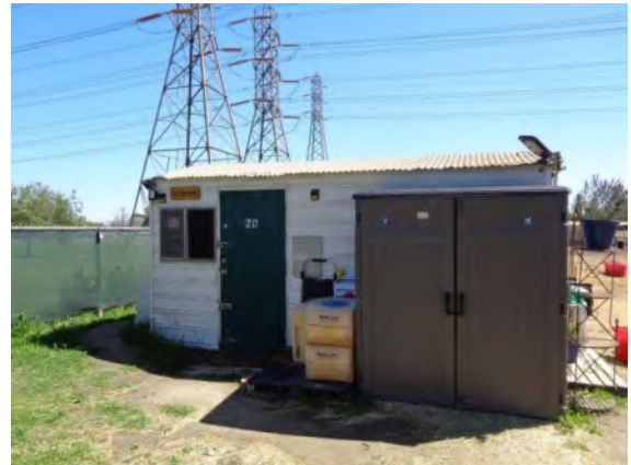
0042120a 4/2/2024 Corrugated metal roof and siding and door with knob hardware Tack shed 20
