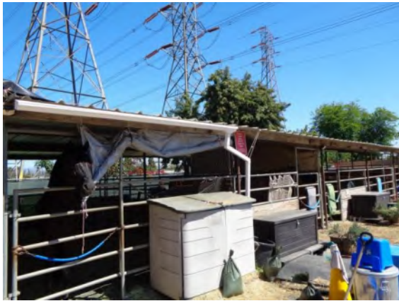
0042094a 4/2/2024 Boarding stalls with corrugated metal roof and pipe rail fencing Stalls 142-146
