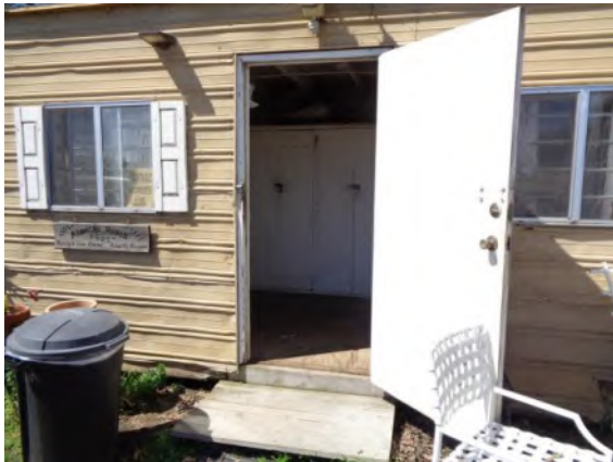
0042119a 4/2/2024 Unfinished wood floor and door with knob hardware Tack shed 21
