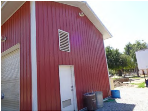
0042061a 4/2/2024 Corrugated metal exterior walls Hay barn, west elevation
