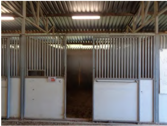
0042034a 4/2/2024 Typical sliding stall door Barn 1-29 interior
