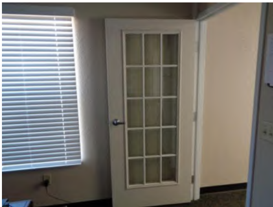
0042005a 4/2/2024 Interior door with glass lites and lever hardware Office
