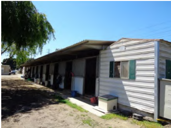
0042050a 4/2/2024 Corrugated metal roof, and sliding stall doors Barn 30-39, east elevation
