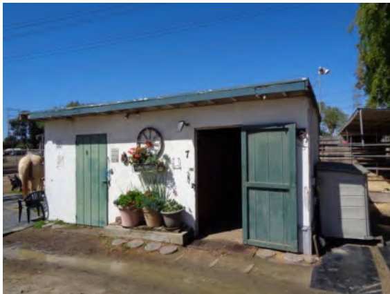
0042121a 4/2/2024 Painted exterior and wood doors Tack sheds 7 and 8
