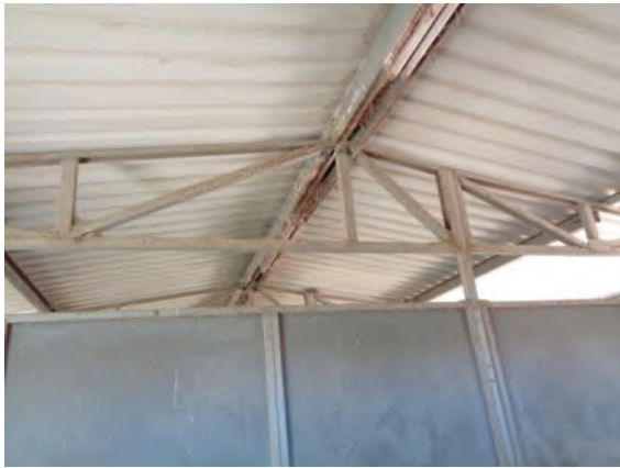
0042052a 4/2/2024 Corrugated metal roof supported on tubular steel frame Barn 30-39, interior
