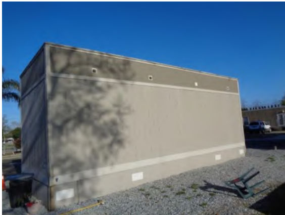
0042026a 4/2/2024 Painted T-111 plywood siding and skirting Restroom building, east elevation
