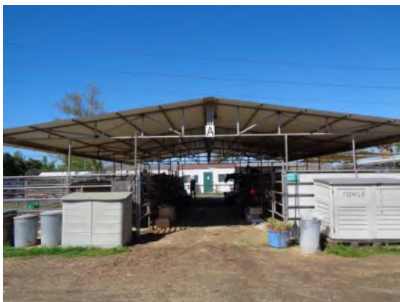
0042090a 4/2/2024 Boarding stalls with center breezeway and corrugated metal roofing on steel tubular frame Stalls 40-46
