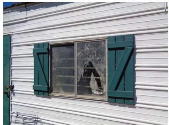
0042116a 4/2/2024 Typical single-pane glass window Tack shed 10
