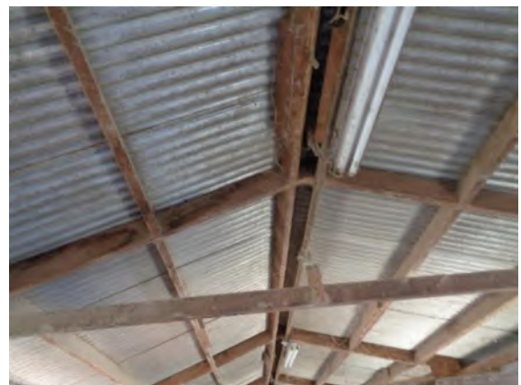
0042104a 4/2/2024 Corrugated metal roof on wood frame Stalls 170-172
