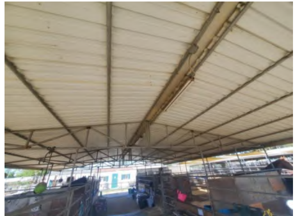
0042074e 4/2/2024 Overview of stall systems Stalls 40-46
