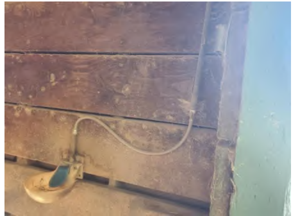
0042034e 4/2/2024 Galvanized steel pipe and steel waterer Stalls 170-172
