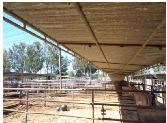
0042098a 4/2/2024 Galvanized corrugated metal roofing and pipe rail fencing Stalls 124-135
