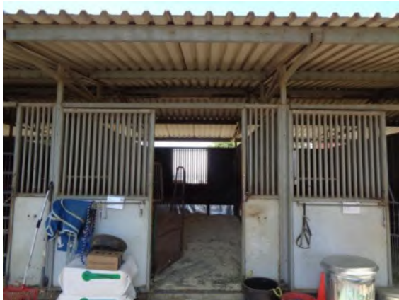
0042054a 4/2/2024 Sliding stall doors Barn 30-39, east elevation
