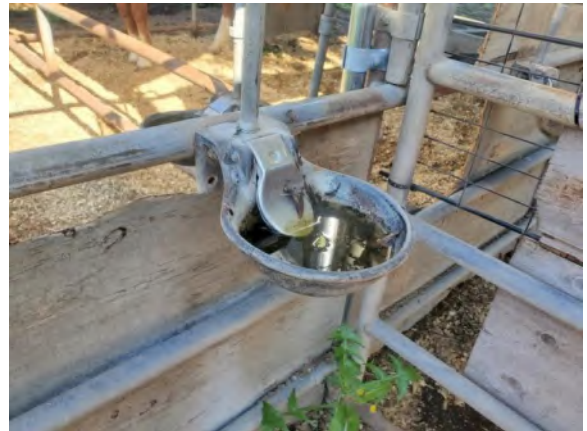
0042050e 4/2/2024 Galvanized steel pipe and steel waterer Stalls 181-188
