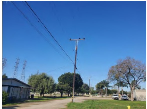
0042049e 4/2/2024 Utility-owned power lines and wooden poles Site
