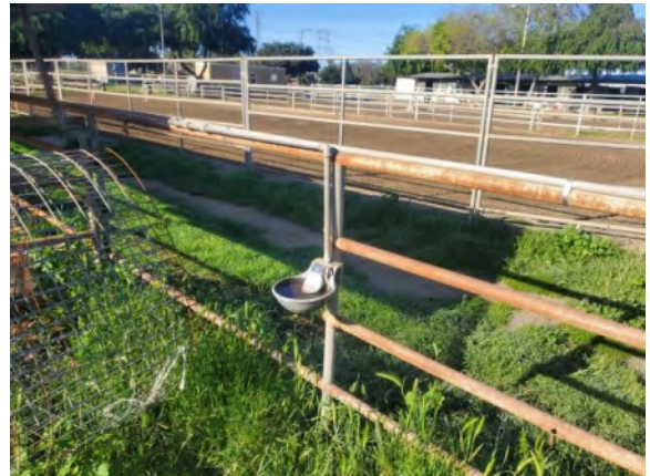
0042031e 4/2/2024 Steel waterer Stalls 152-158
