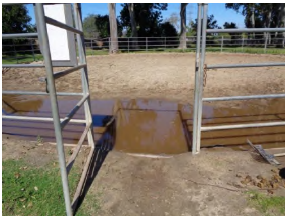
0042133a 4/2/2024 Standing water Turnout 6
