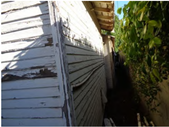
0042111a 4/2/2024 Wood siding on rear wall Tack shed
