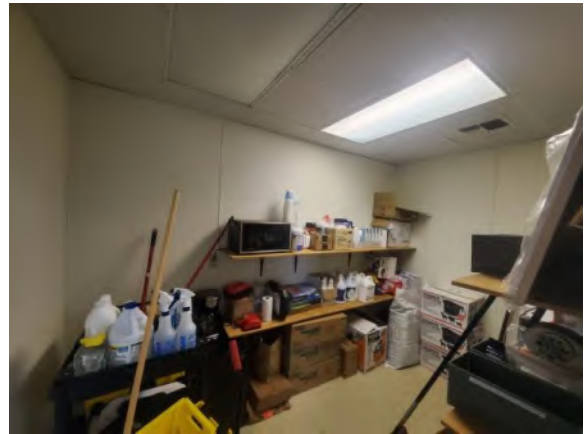
0042022e 4/2/2024 Overview of storage area systems Office, storage room
