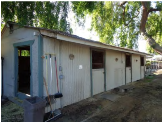
0042101a 4/2/2024 Enclosed boarding stalls with corrugated metal roof, wood siding, and corrugated metal siding Stalls 170-172
