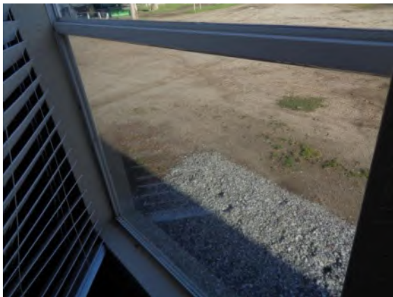
0042003a 4/2/2024 Window with single-pane glass Office
