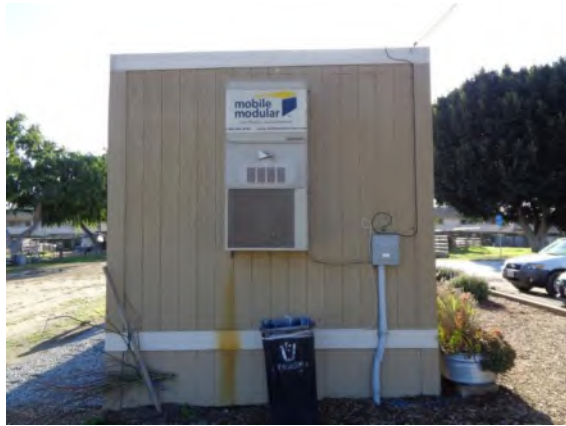
0042010a 4/2/2024 Painted T-111 plywood siding and skirting Office, west elevation
