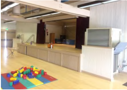
new lift and accessible stair retrofit At Heritage Park Community Center
