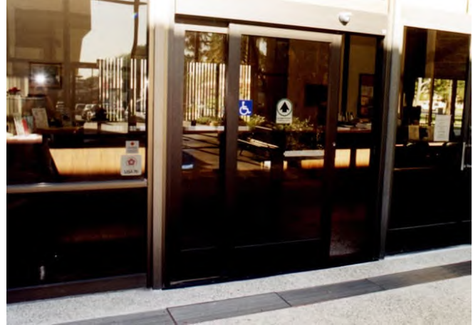
New automatic doors to main entry to City Hall
