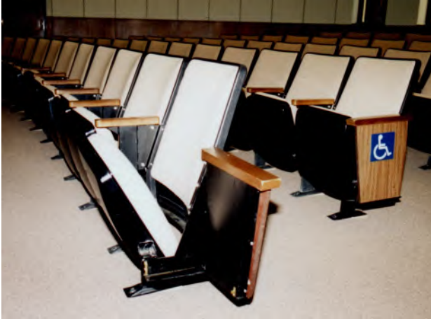
New fixed seating and new semi-ambulatory seats.
