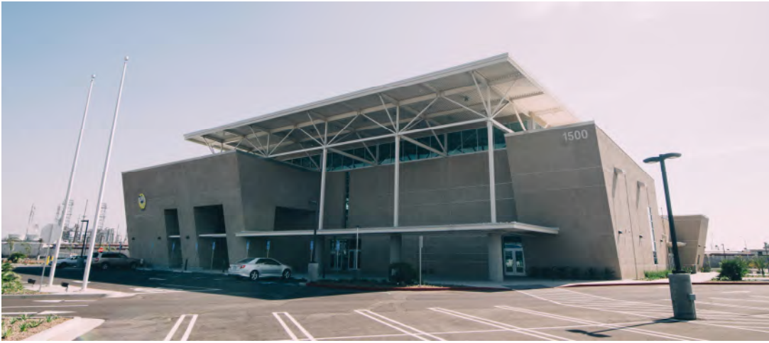
ILWU Dispatch Center main entry
