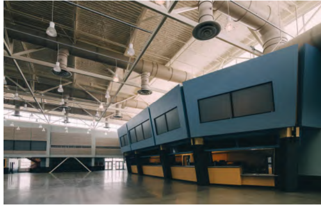
Dispatch Hall with 14 large high definition 10'x7' rear-projection screens
