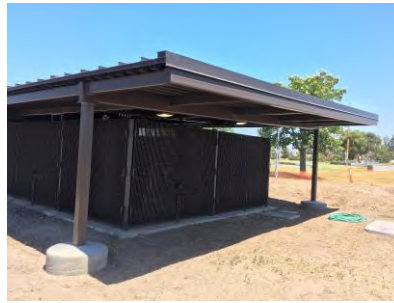
new roof structure over pump equip. At Great Park Pump Station, 2018
