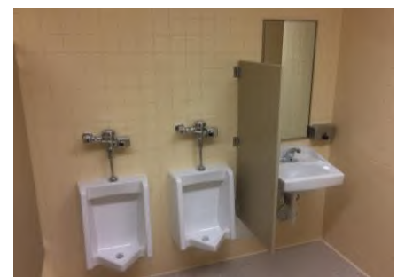
new accessible restroom
